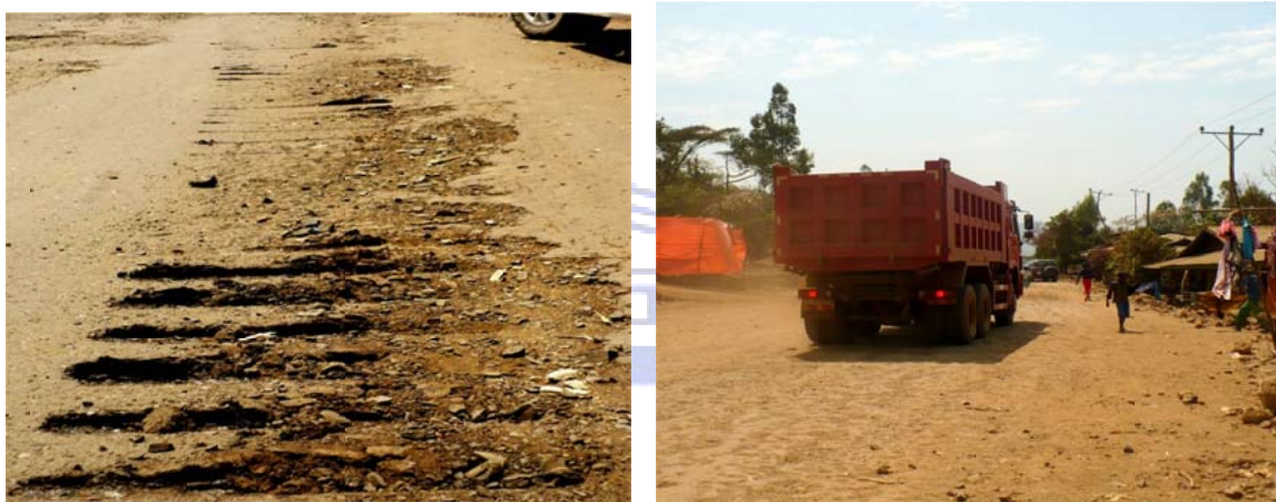
Figure 6.2: A primary road in Wutete village potholed by trucks of the COFCOP
