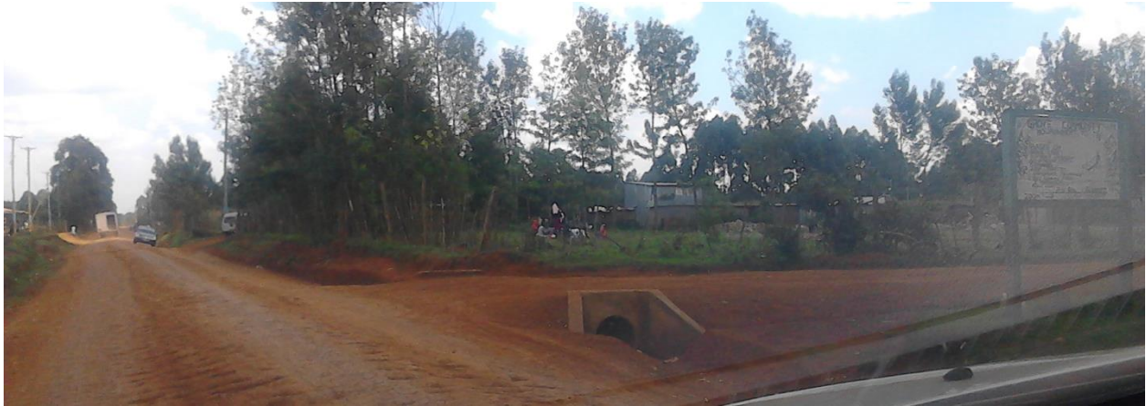
Photo 6: Photo showing the absence of zebra crossing in a road intersection in rural area.
