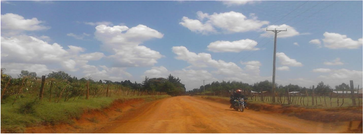
Photo 3: Road showing absence of sidewalks rural area
