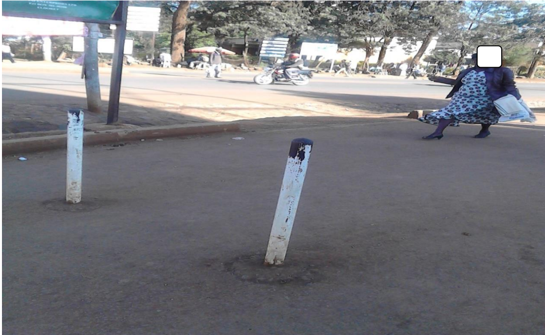
Photo 5: Photo showing sidewalks in urban area
