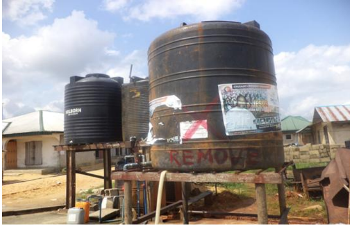
Picture source: Authors picture; the rusty borehole drinking water tank in Amasoma community
