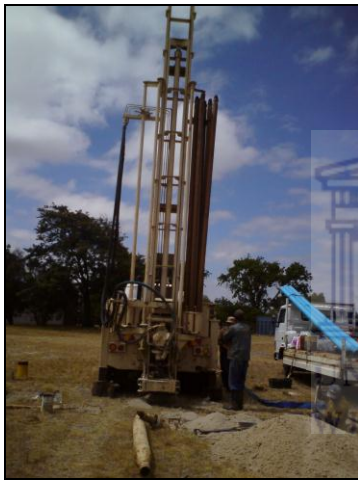
c) Mud rotary drill rig
