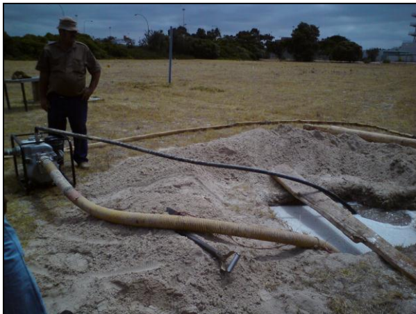
e) Removal of drilling cuttings by pumping fluid
