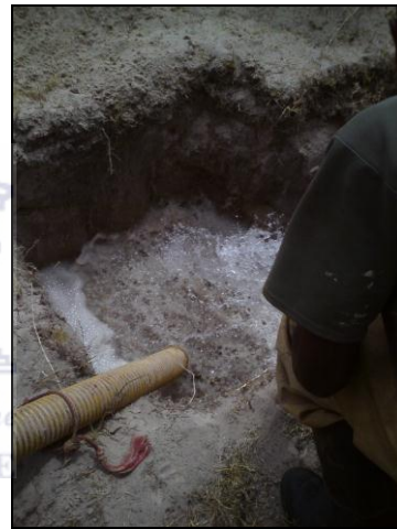
d) Pumping fluid added to stabilize borehole walls
