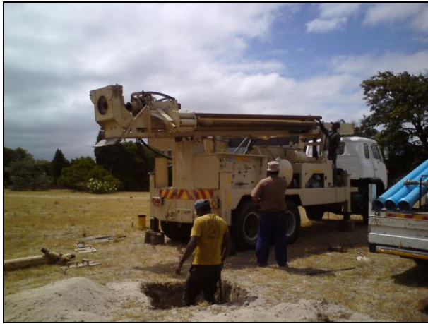
a) Preparation of the hole
