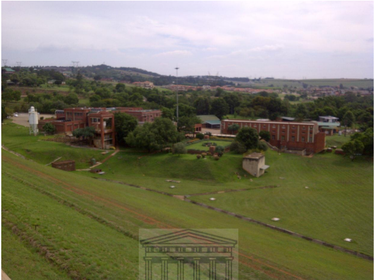
The Rietvlei Water Treatment Works buildings. The dam is on the left of this picture. Source: Author (2011)
