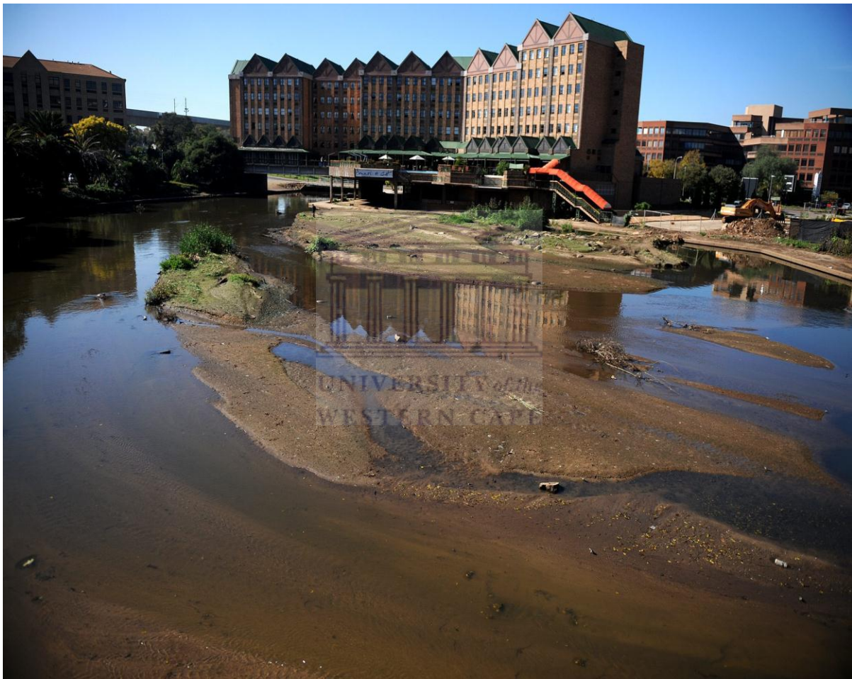
Silt filling up the lake area. Source: Pretoria News
