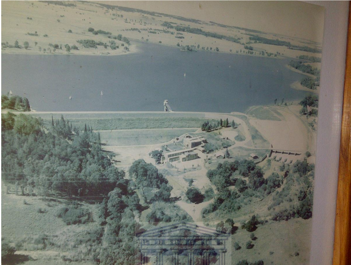
Aerial photo of the Rietvlei Dam. The treatment works can be seen in front of the bushes. It receives water from the dam via a short underground pipe. Source: Author (2001). Photo adapted from an old photo owned by the City of Tshwane.
