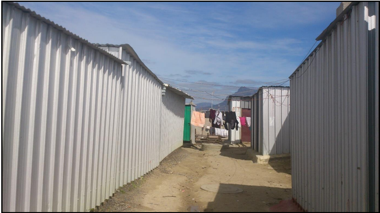
Figure 35: Mshini Wam: Re-blocked structures Source : Sibanda (2015)
