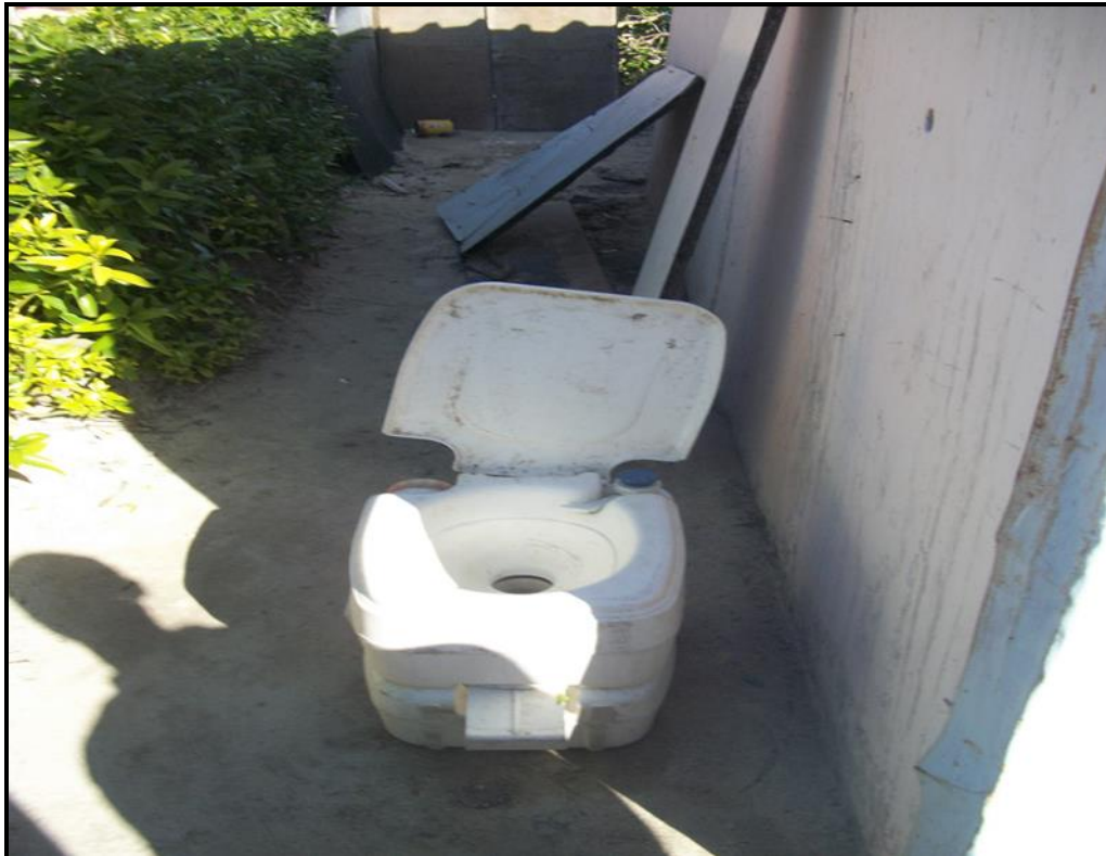
Figure 33: Portable flash toilet in Nkanini Source: Sibanda (2014)
