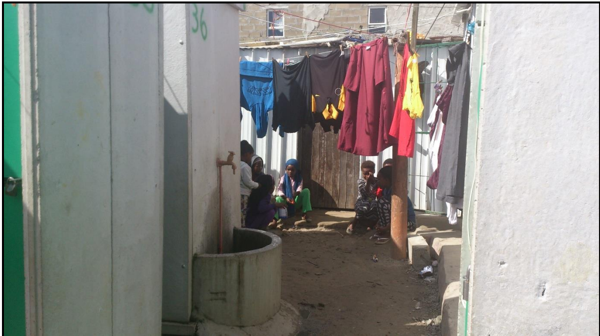
Figure 34: Mshini Wam: Water and sanitation services after re-blocking Source: Sibanda (2015)
