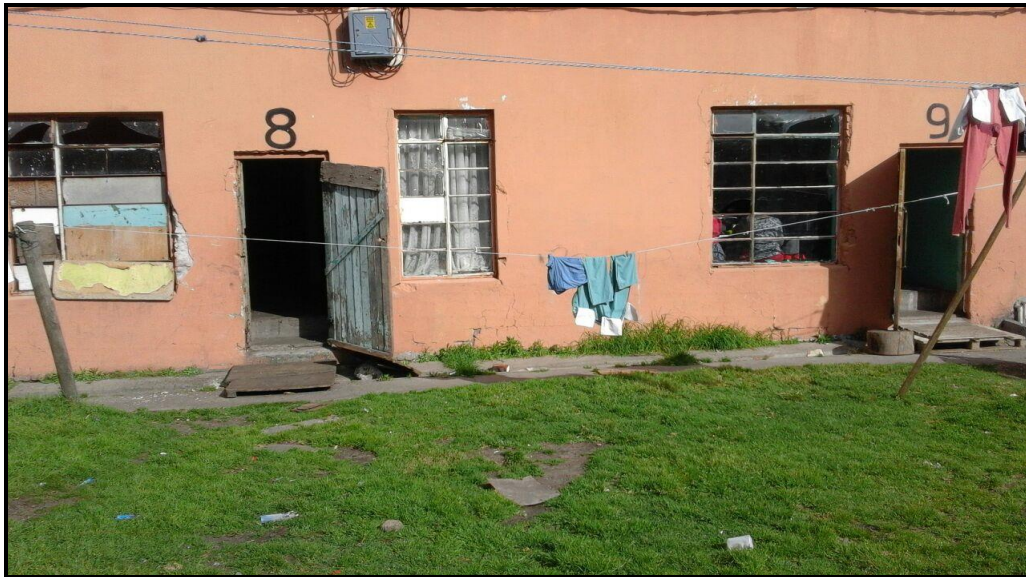
Figure 24: Langa Old Hostels Source: Sibanda (2015)
