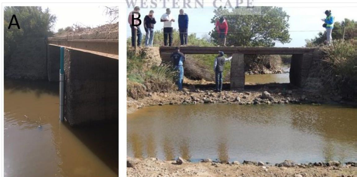
Figure 4.25: Stilling well installed at Elandsdrift (A) and the Elandsdrift bridge during the selection of the flow monitoring site in 2014 (B).
