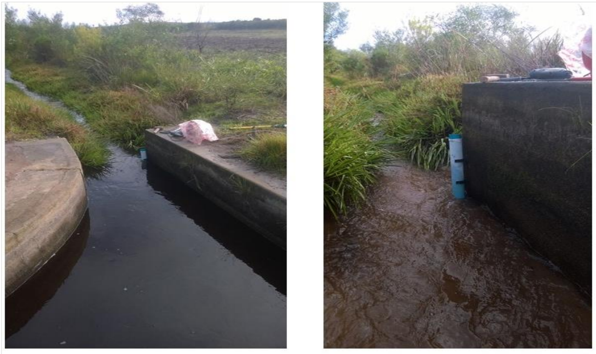
Figure 4.22: Flow measuring site along the Upper Nuwejaars River at the Elim Flow Diversion.
