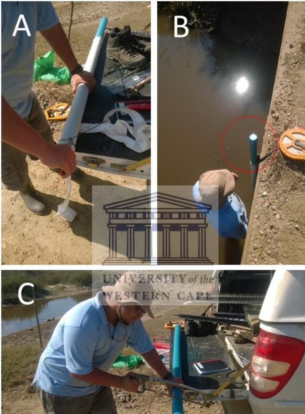
Annexure 2: Fabric mesh (A), PVC cap and 14 mm bolt with lock-nut (B), and slits being cut into the 75 mm PVC pipes used as stilling wells (C).
