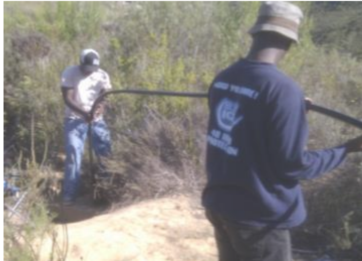
Figure 4.2: Insertion of PVC injection pipe into BH5
