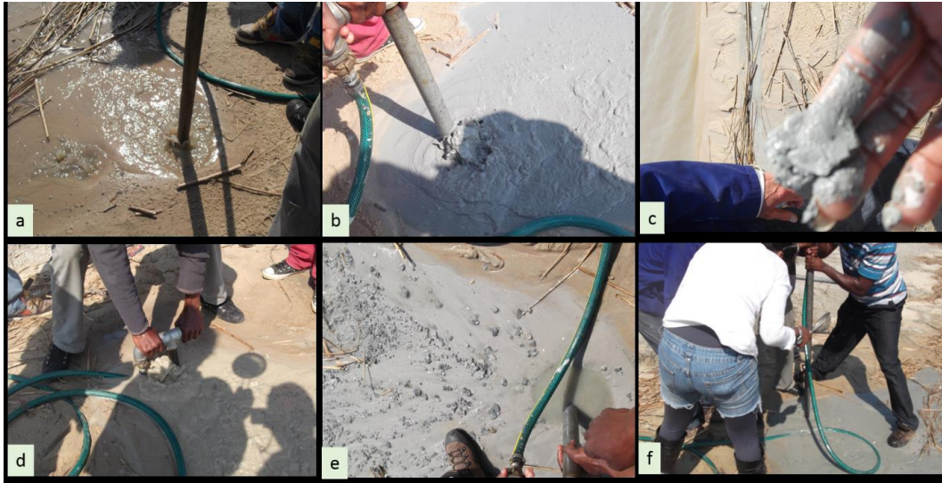
Figure 4.7: The figure shows the hydraulic injection at the Voelvlei site.
