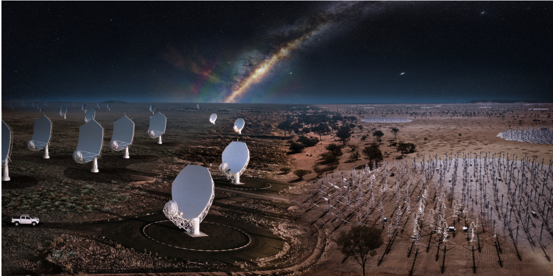
FIGURE 1.9: An artistic composite image of the SKAO telescope, comparing the different radio telescopes to be hosted at its two major sites. On the left are the mid-frequency dishes in the upper Karoo desert of South Africa and on the right are the frequency dipole antennas of the SKAO low-frequency array at the Murchison Radio Observatory in Western Australia (From: https://www.skatelescope.org/the-ska-project/ ).
