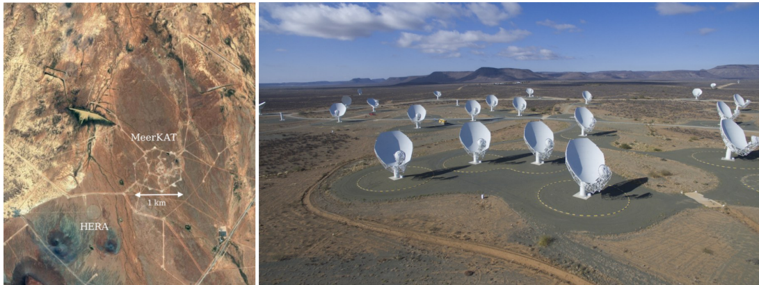
FIGURE 1.10: On the left is a Google Earth satellite view of the inner core of the MeerKAT foundations prior to installation. The type of distribution is dependent on the type of science the MeerKAT radio telescope will perform. On the right is a wide view of the MeerKAT dishes shown to illustrate the design of the dishes (courtesy: Asad et al. [2021]).
